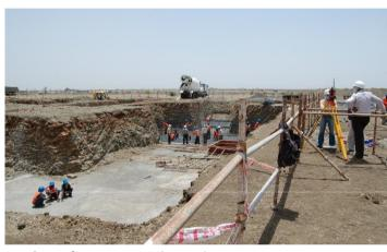
PCC & Reinforcement Work in Boiler Unit 1
